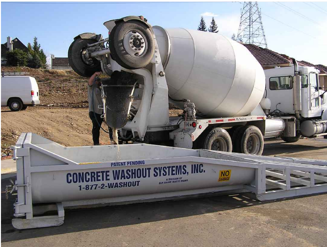
3 TEMP. CONCRETE WASHOUT NOT TO SCALE
