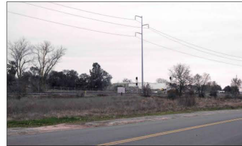
In their 2001 report, PG&E prepared simulations of how the powerline would look if installed. It would carry 65,000 kilovolts, but would be built to 115,000 kilovolt standards to allow for future expansion. Above is the view from Railroad Ave. which today includes the train depot, Old St. Mary's, and Heritage Park. The view below is Front Street, looking toward the firehouse and the community orchard.
