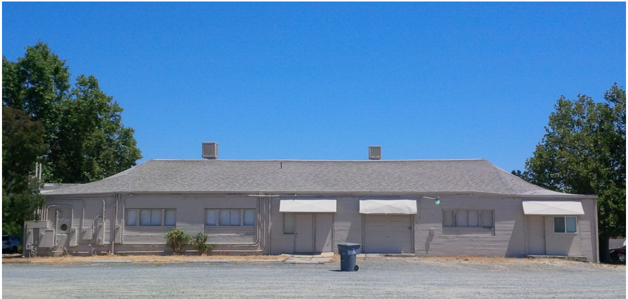
2 - Side of the building looking east
