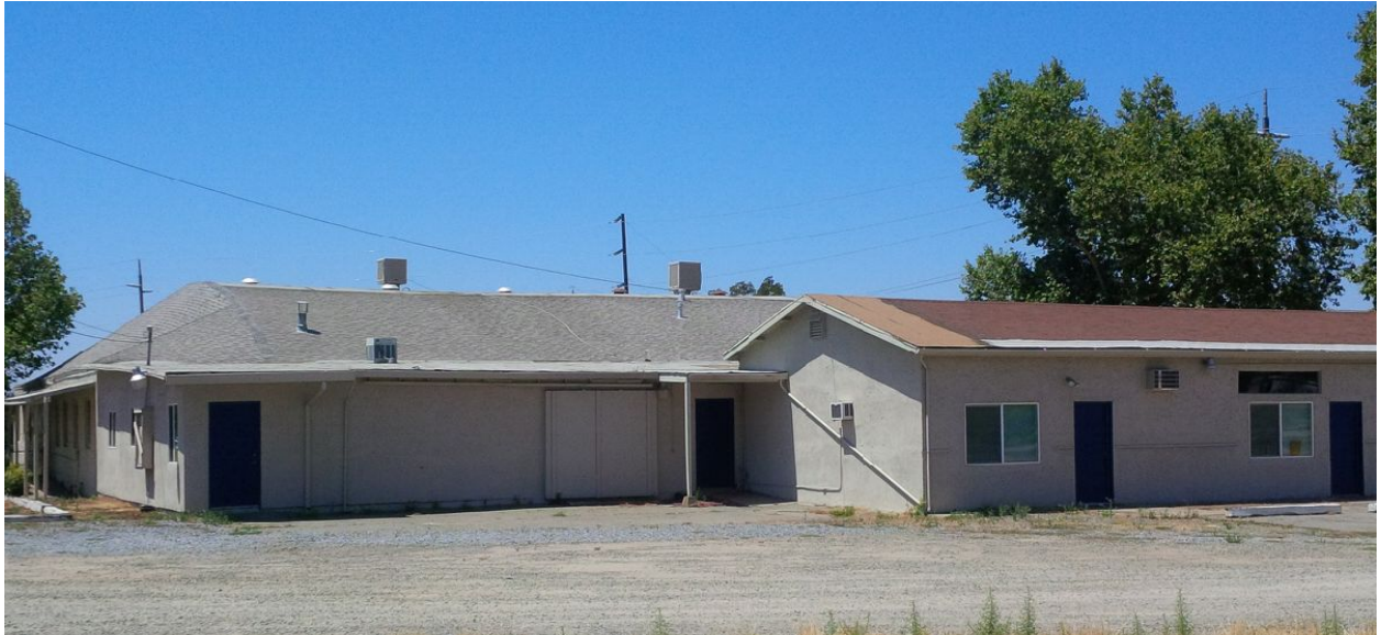
3 - Side of building looking west
