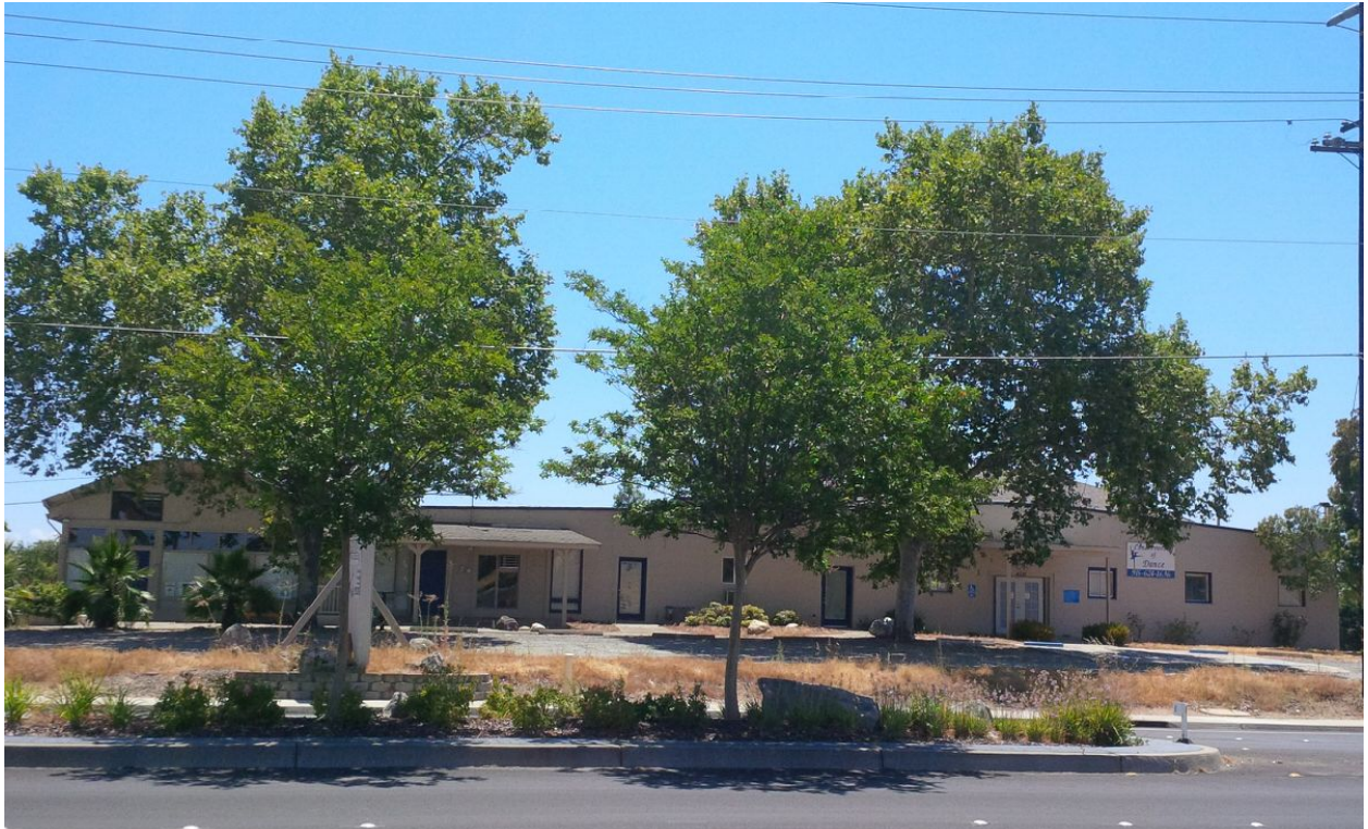
1 - Front of the building looking south
