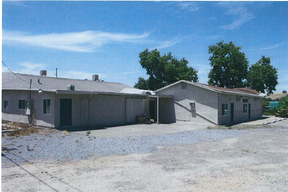
Figure 10: View looking west at the rear and side additions, evidenced by wood-frame and stucco-clad construction. The original domed-shape Hall can be seen to the left rising above the flat-roofed extension.
