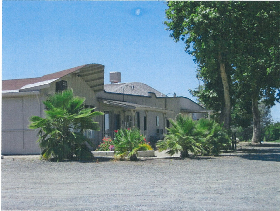
Figure 7. North elevation of Pleasure Hall/Stardust Skating Rink building at 4545 Pacific Street.
