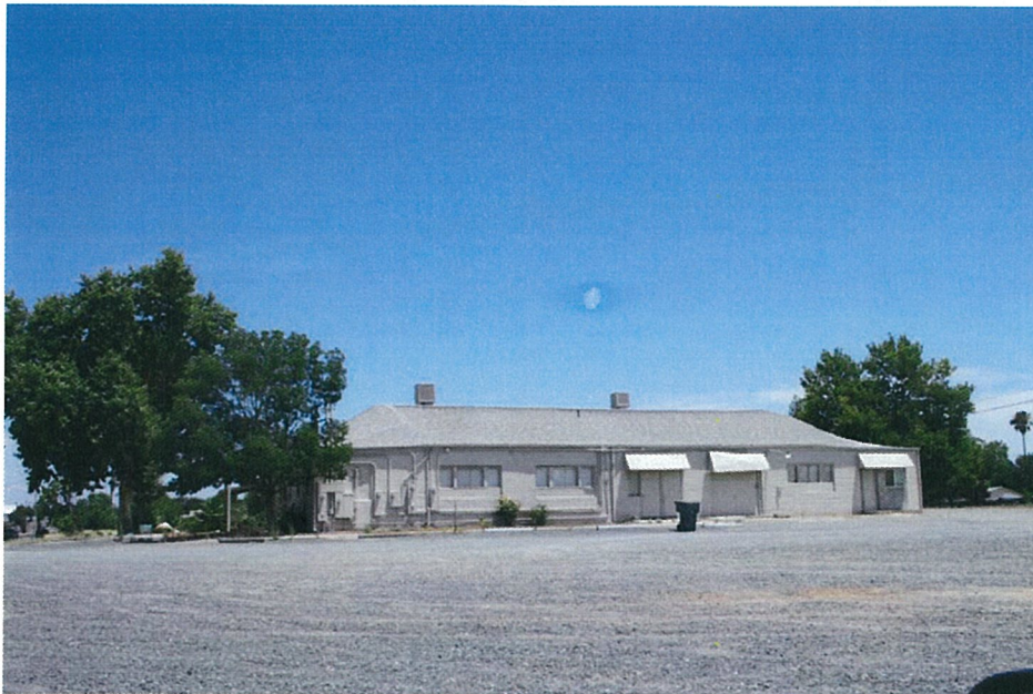
Figure 8: Southeast side elevation of the property, looking northeast.
