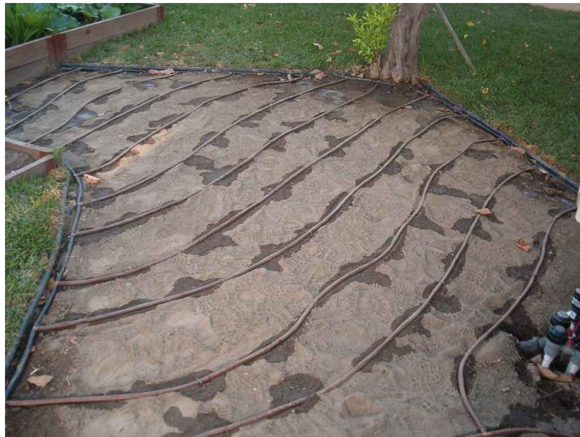
SUB-SURFACE DRIP IRRIGATION
