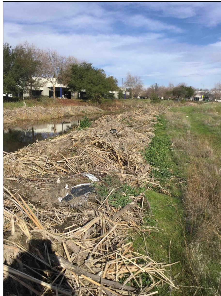
Dredged material deposited on east bank of Creek; Looking North. Photo Date: January 27, 2020.
