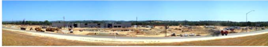
Rocklin Crossings Under Construction - Sierra College & Interstate 80
