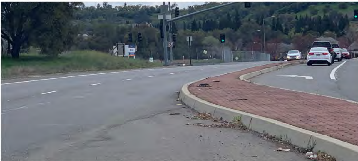
Image 3:View from original left-turn lane location serving retail center (looking south toward Rocklin Road).
