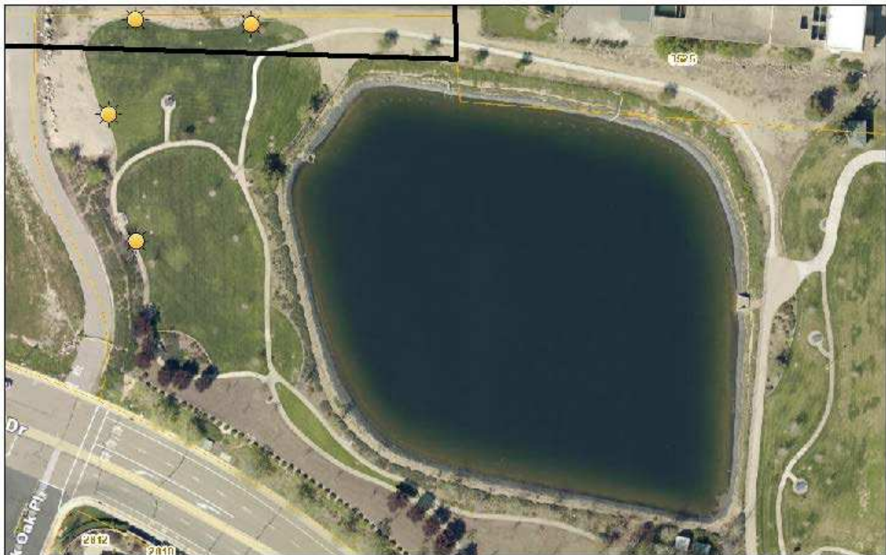
Boulder Ridge Lighting Addition
