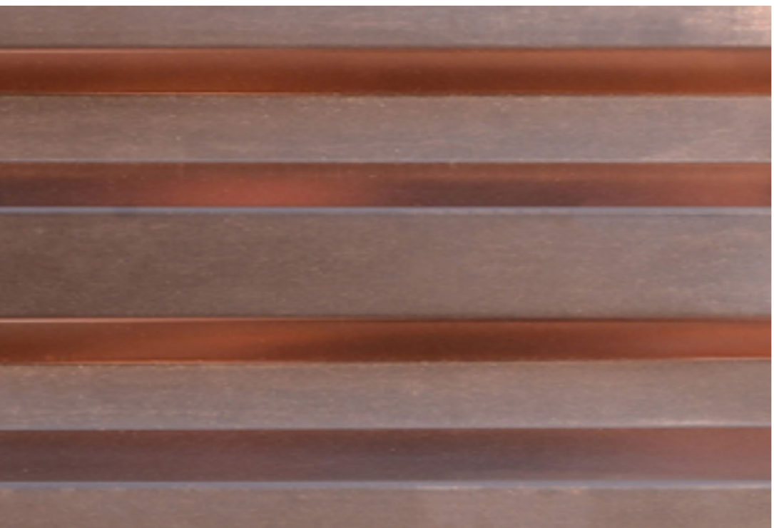
METAL PANEL AT BUILDING: WESTERN STATES METAL - WESTERN WAVE 24 GA. ORIENTATION: VERTICAL
