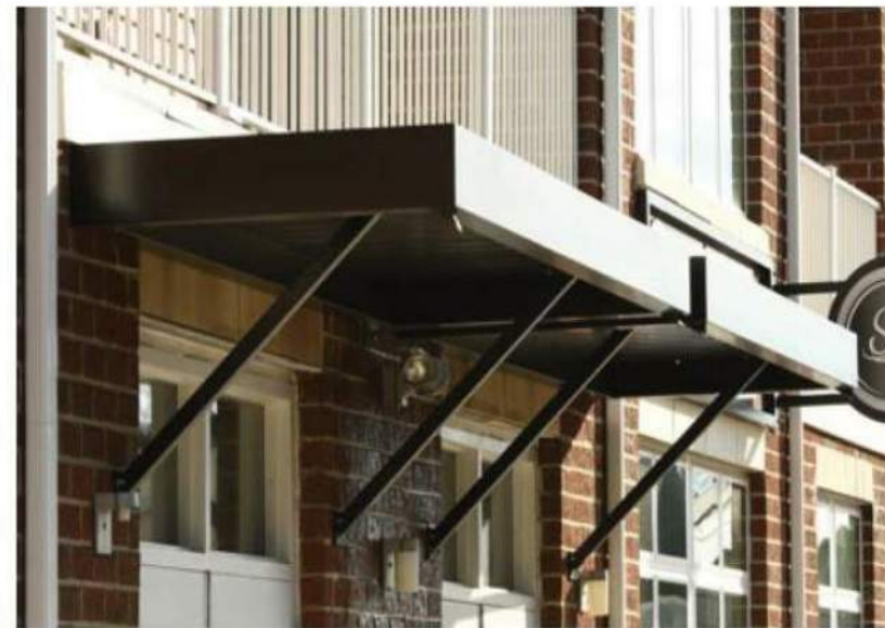
METAL CANOPY WITH CORBELS
