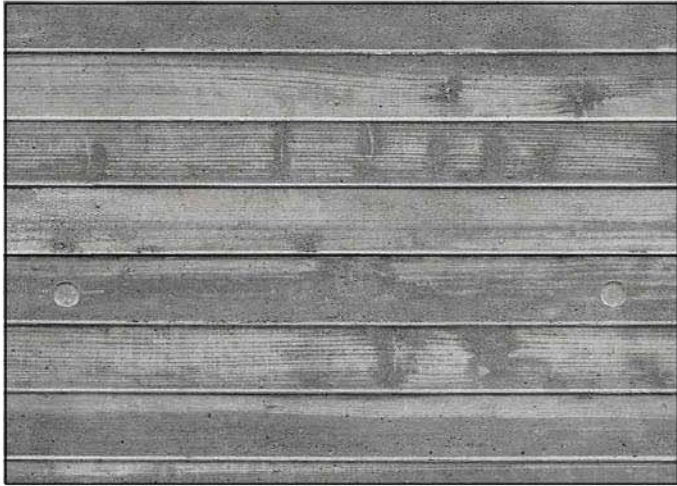
BOARD FORMED CONCRETE
