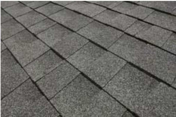
ASPHALT COMPOSITION ROOF
