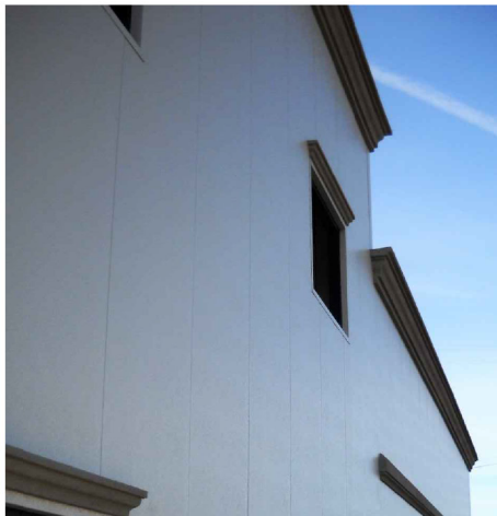
INSULATED METAL PANEL AWIP - ADOBETEXTURE (HE40A) PAINTED TO MATCH EXISTING CENTER
