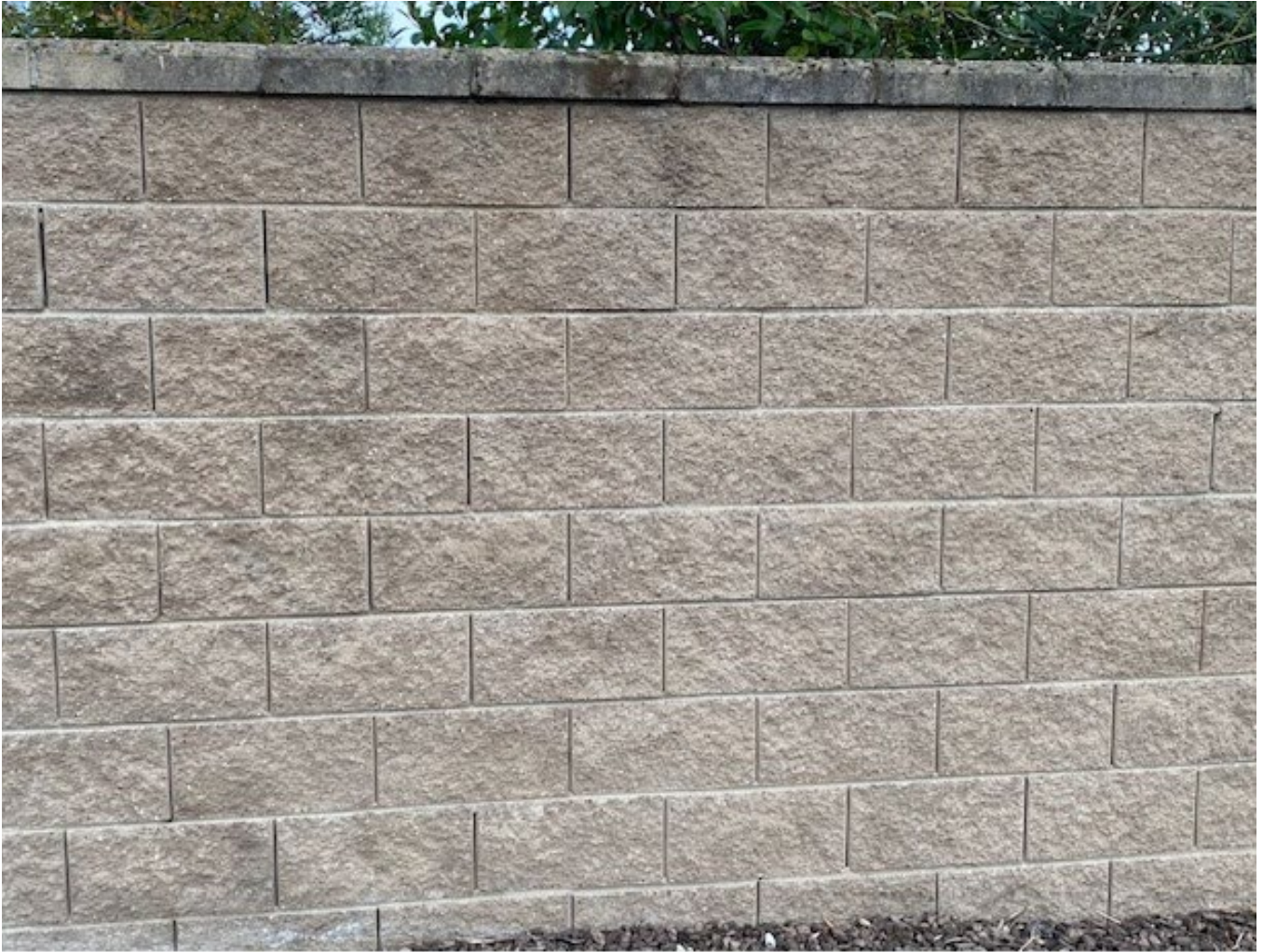
Example of a typical City of Rocklin Proto Wall and cap.
