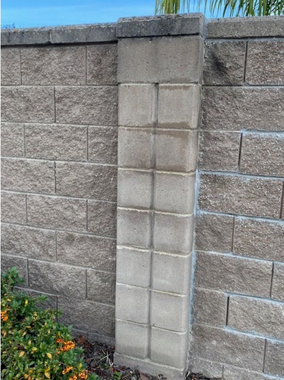
Example of a 6 foot wall column
