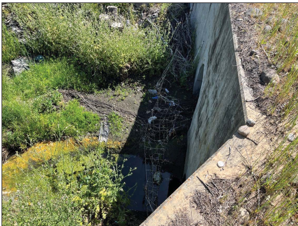
Old fencing and trash in culvert mouth, Sunset West (SW-8) | May 23, 2023 (L. Neuhaus)
