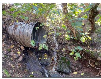
Rusted out culvert outlet within Stanford Ranch (SR-15). Flow emerges from underneath pipe.
