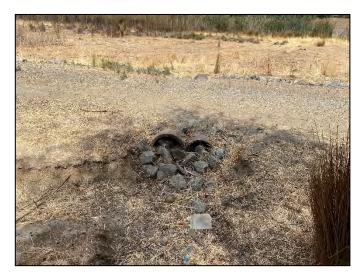
View of plugged culvert within Sunset West (SW-3) where a small diversion channel was dug by hand upstream.
