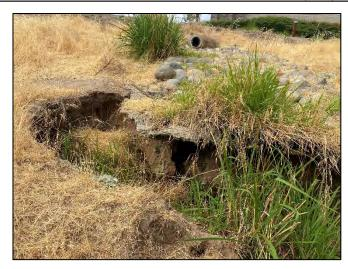
Erosion site within Sunset West (SW-4) where a gully is forming, and an armored outfall is being undermined.
