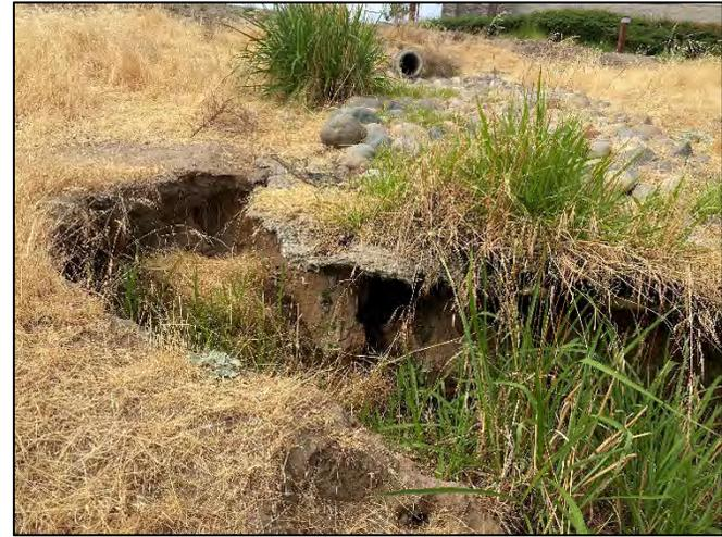
Erosion site within Sunset West (SW-4) where a gully is forming, and an armored outfall is being undermined.
