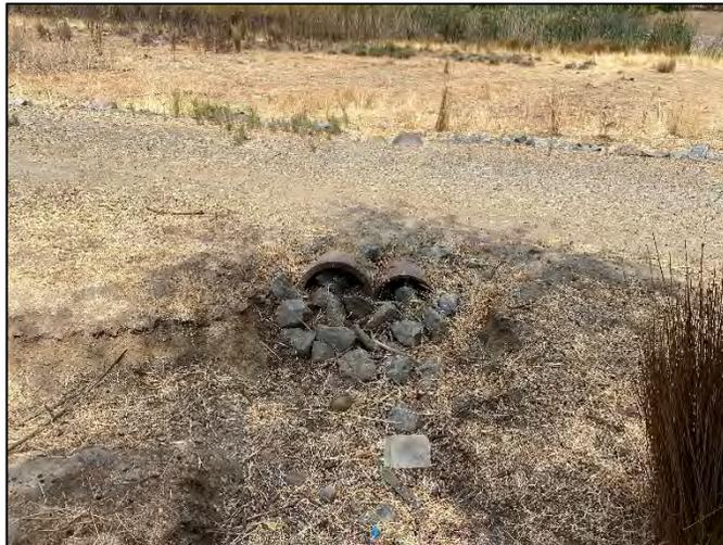
View of plugged culvert within Sunset West (SW-3) where a small diversion channel was dug by hand upstream.
