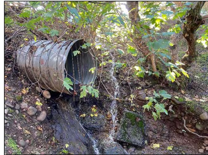
Rusted out culvert outlet within Stanford Ranch (SR-15). Flow emerges from underneath pipe.
