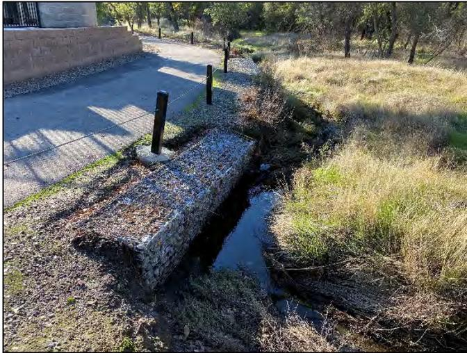
Erosion site within Garnet Creek. Gabion basket is being undercut by creek and is slumping.
