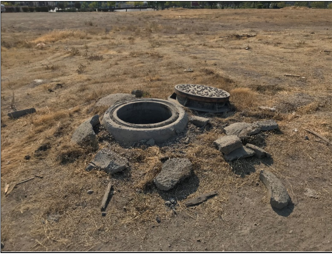
13. Sewer utility manhole located on-site
