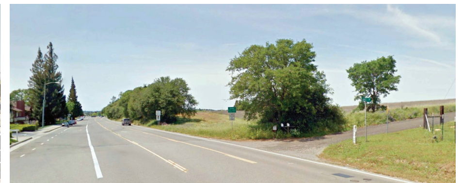
① VIEW FROM ROCKLIN ROAD
