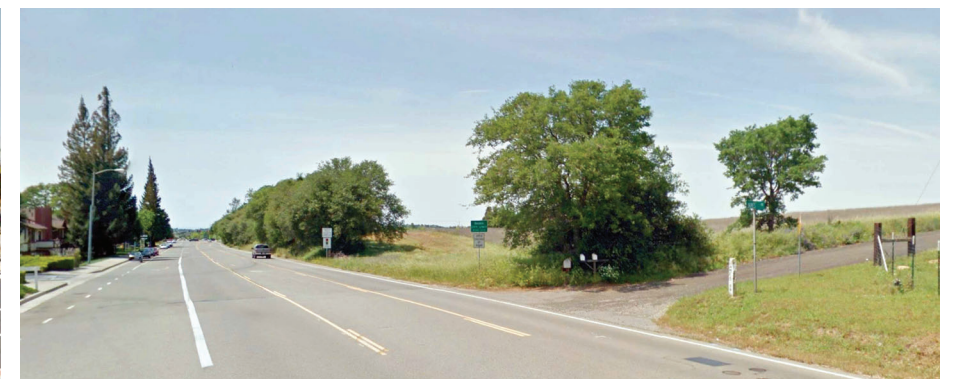
① VIEW FROM ROCKLIN ROAD
